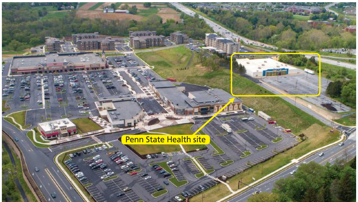
An aerial photo of The Crossings at Conestoga Creek shows the former Toys R Us store in the upper right next to the Residence Inn by Marriott.
